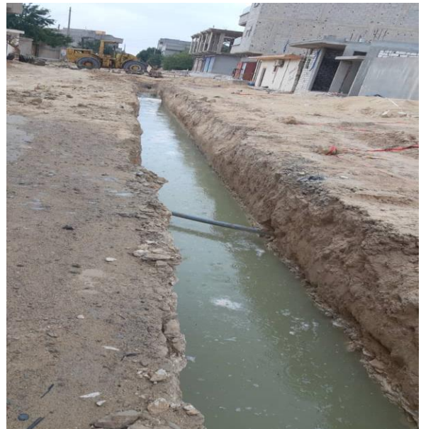
Fig. 5 Rising water table during maintenance operations.
