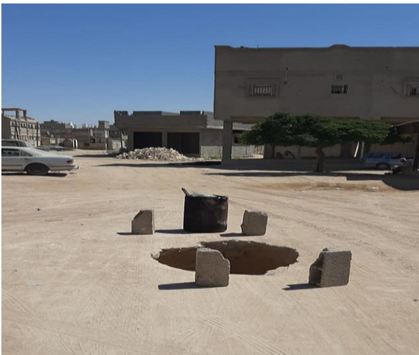
Fig. 12 Pictures of some of the subsidence and sinkholes in the city
