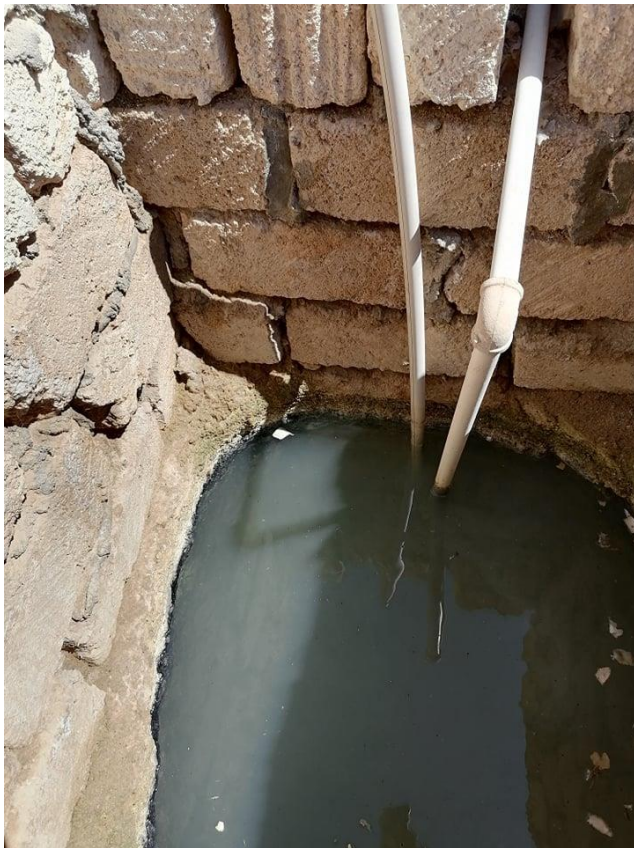
Fig. 9 Groundwater pollution with the sewage water
