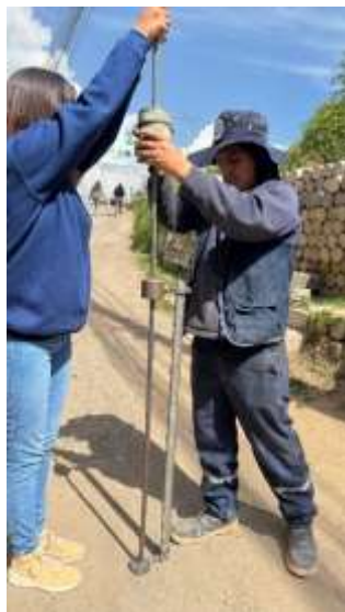
Fig. 5 Dynamic Cone Penetrometer test (DCP) to evaluate the strength of the soil in its natural state
