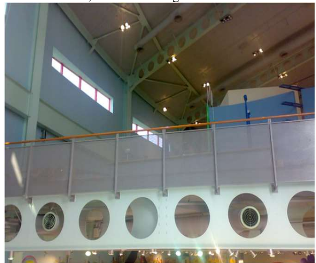
Fig. 3 Cellular Beams Can be Used to Build Different Components of a Structural System [6]
